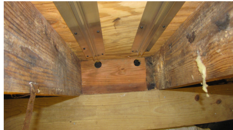
Joist Trak plates for 1/2" PEX tubing
